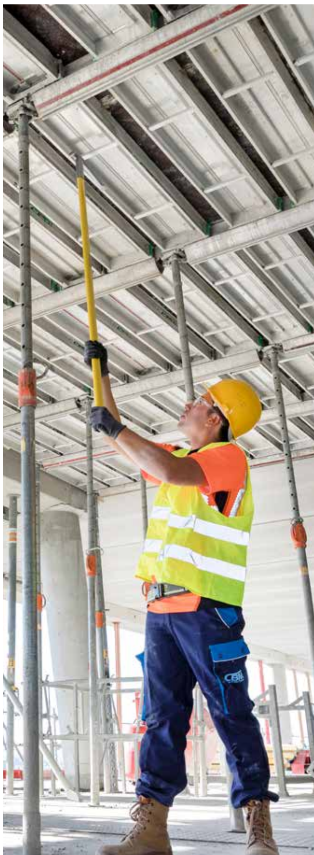
Long-range form stripping tool in use
